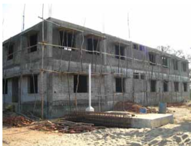
Construction of the Resource Center
